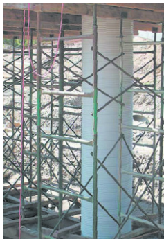
Column supported by Soffit formwork
