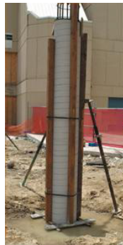
Freestanding column braced and propped
