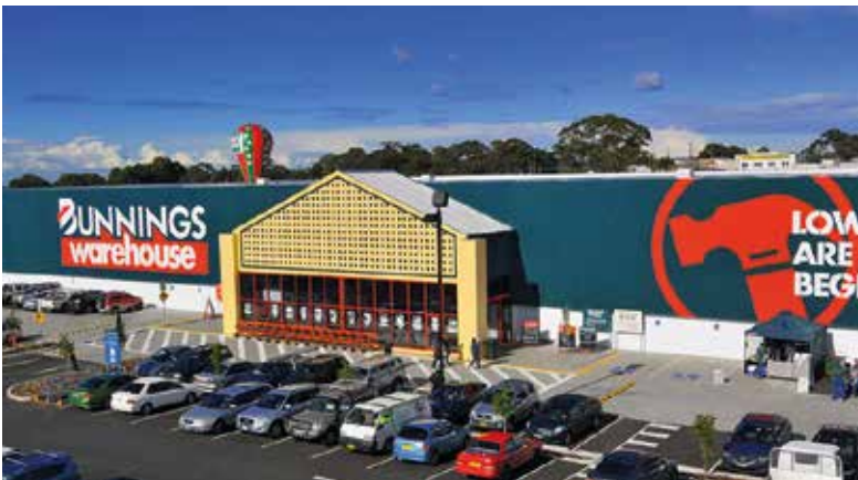
Bunnings Warehouse SYDNEY, AUSTRALIA
